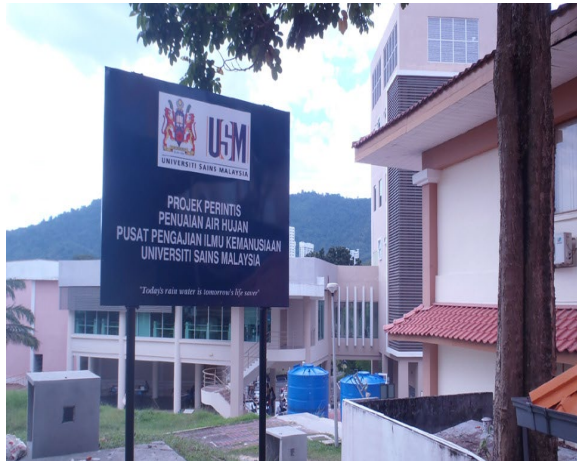
The location signage for one of the rainwaters harvesting system
