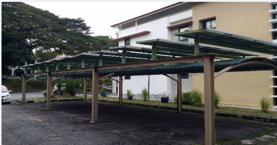
SOLAR PARKING LOT (2.0 Kwh)- -Solar Power
