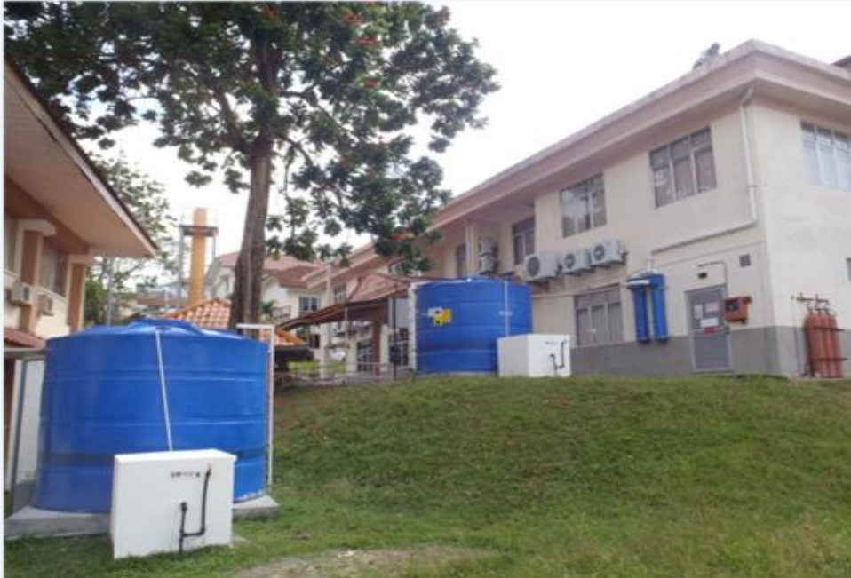
Rain harvesting system installed in campus
