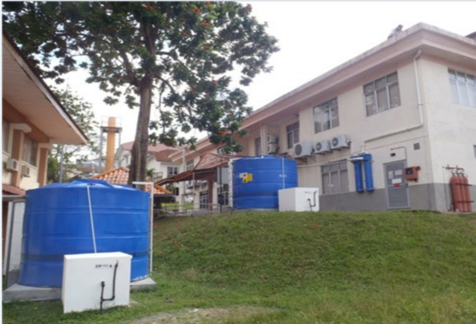
Rain harvesting system installed in campus
