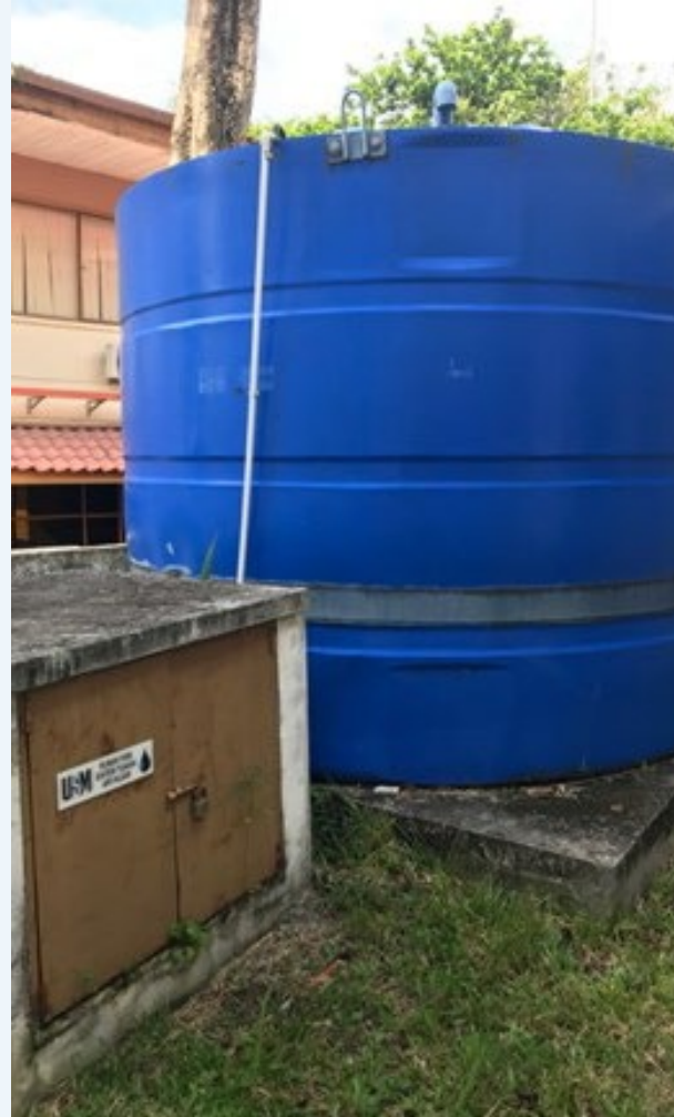
Rain harvesting system installed in campus
